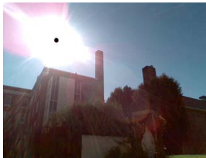
E Falling Hazard
