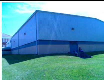
NE Elevation View
