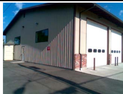
SW Elevation View
