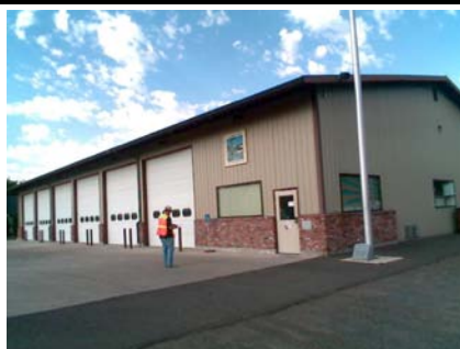
NE Elevation View
