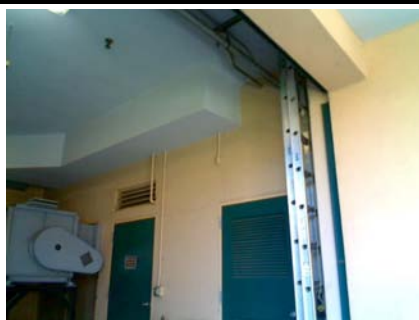
S Primary Structural Type basement
