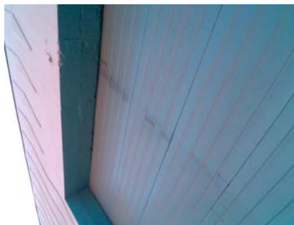
N Primary Structural Type wall about 12" thick
