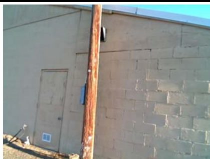
S Building Quality lean-to addn poor masonry
