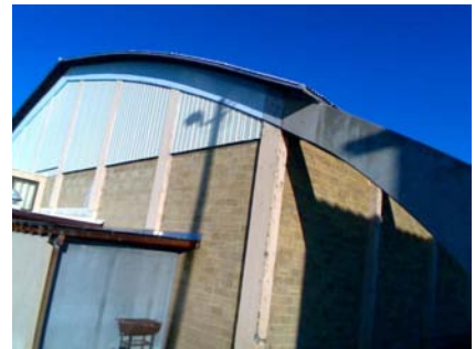
SE Primary Structural Type 3 hinged arches and buttresses
