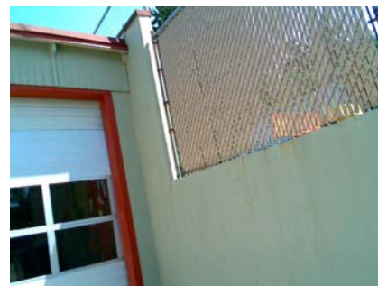
SW Secondary Structural Type concrete retaining wall on East side
