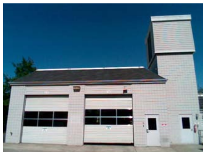
SW General Site Tower is RM1
