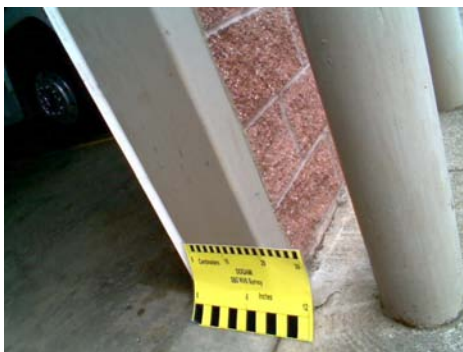
NE Secondary Structural Type ~1/8 thick U-channel frames garage doors. RM1 walls appear to only go up 4.5ft and don't appear to con
