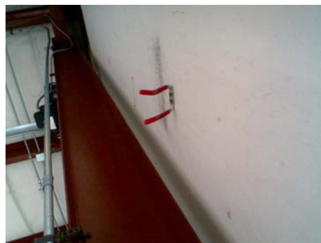
NE Primary Structural Type steel column does not appear to tie in to the wall. View is looking up the wall.
