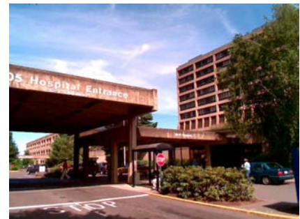
SE Pounding Potential over main ent
