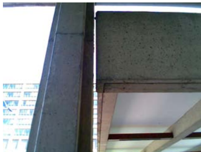
S Pounding Potential out of plain elements are separated by ~1".
