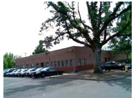
NW General Site
