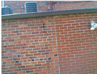
E Primary Structural Type older URM on left.
