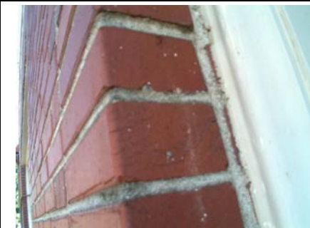
W Primary Structural Type second layer of brick just visible near window frame.
