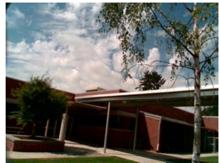
NW Falling Hazard
