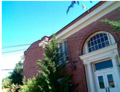
SW Falling Hazard Heavy Cornice
