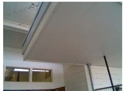
N Falling Hazard covered walkway, 6 foot cantilevered. roof shows ~8" of sag on side nearest school door
