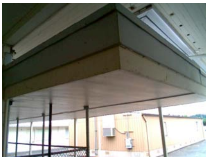
SE Falling Hazard covered walkway, 6 foot cantilevered. roof shows ~8" of sag on side nearest school door
