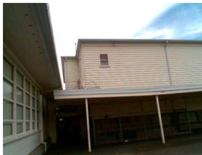
NW Falling Hazard covered walkway, 6 foot cantilevered. roof shows ~8" of sag on side nearest school door
