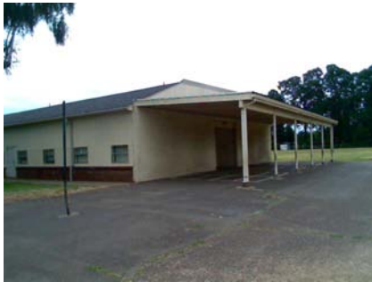
SW Falling Hazard
