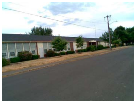
NW General Site
