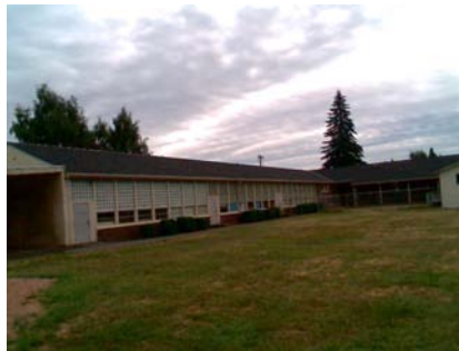
NE General Site
