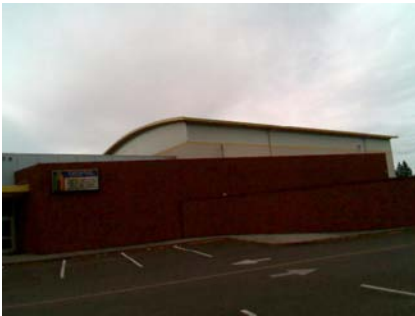
SW General Site
