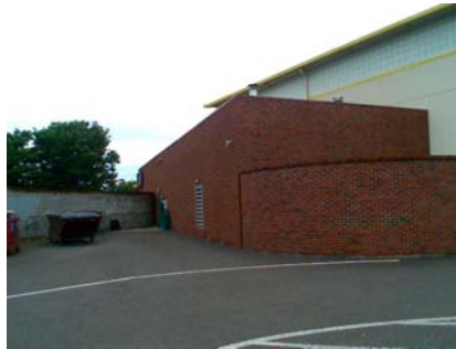
NE General Site kitchen no RVS
