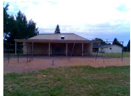
NE General Site
