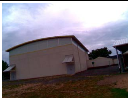
NW General Site
