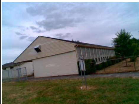
NW General Site
