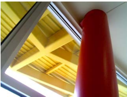
NE Primary Structural Type roof beams are welded to steel columns
