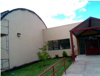
N Pounding Potential Bldg B on left and Bldg A on right
