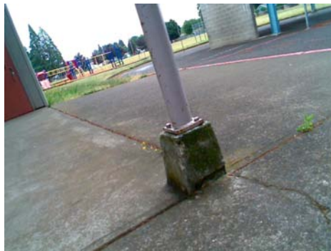
NW Falling Hazard weak connection
