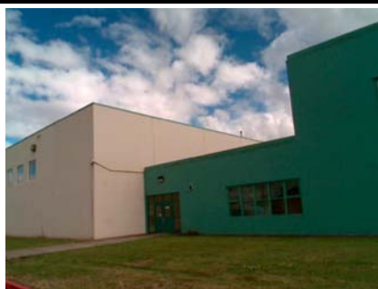
NW Pounding Potential bldg E on left bldg D on right
