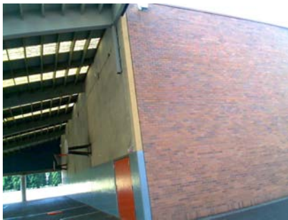
NW Plan Irregularity Primary confirmed W2 with brick veneer on right. Tilt upon left.
