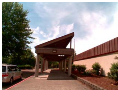
NW General Site
