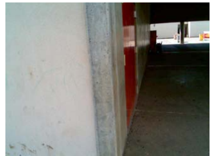
NW Primary Structural Type PC1 on right side W2 on left.
