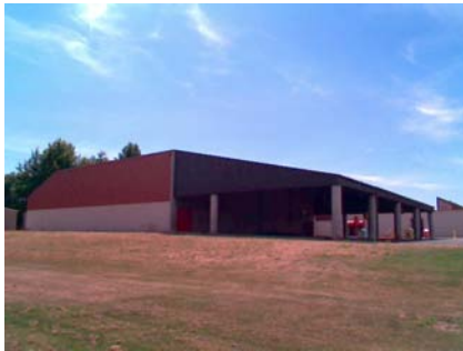
NW General Site
