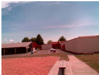
NW General Site
