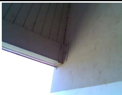
NE Falling Hazard weak connection to covered play area. 6 nails visble
