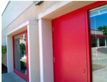
N Falling Hazard Precast Concrete over doorways
