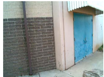
SE Pounding Potential pounding between bldg B and C also out of plane
