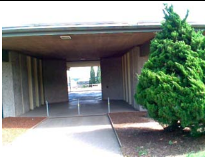
SW Pounding Potential building is broken up in middle
