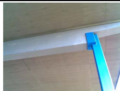
SW Falling Hazard 5in of wooden roof beam rest on column. Bolt may not go all the way through?
