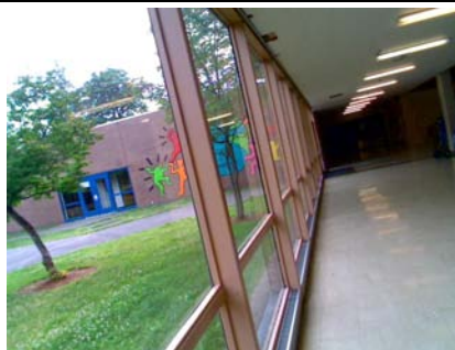
S Secondary Structural Type Steel box tubing 3" x6" on outer walls.
