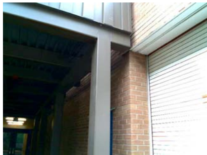
N Pounding Potential Pounding potential on bld B
