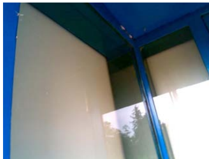
E Primary Structural Type windows and doors framed in with heavy steel box tubing
