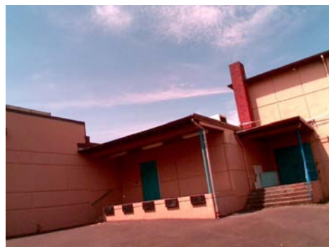
SE Pounding Potential PC1 loading dock against C2. Loading dock addition not RVSe'd.
