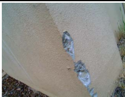
SE Primary Structural Type concrete behind stucco
