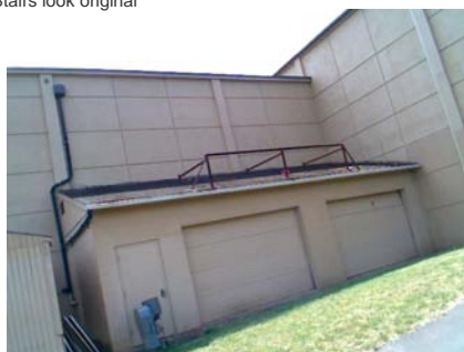
N Pounding Potential RM1 storage against C2.... RM1 not RVSe
