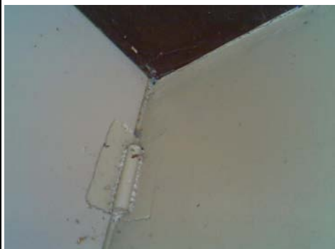
E Building Quality welded joint on PC1 loading dock
