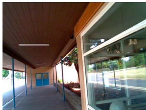
SW Pounding Potential covered walkway connected to building at different edges
