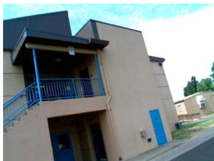
E Pounding Potential RM1 elevator bldg ....pounding On Plan view no RVS. Stairs look original
