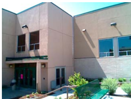
N Building Quality 8in Seismic joint between bldg F and bldg E
