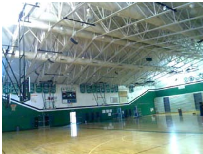
SW Primary Structural Type RM1 on three and one half walls C2 on left side from scoreboard to corner. The rest is RM1
