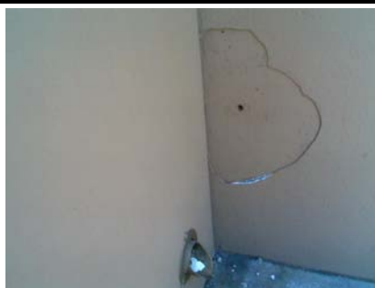
E Primary Structural Type tie rod cone hole
