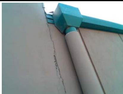
SW Poor Condition cracks between K and M
