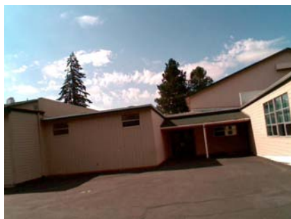
NW Pounding Potential connecting hallway between bld B,C and D
