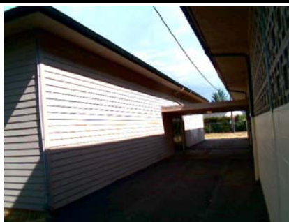
E Pounding Potential covered walkway between bld E and RM1 playarea (not RVSeid)
