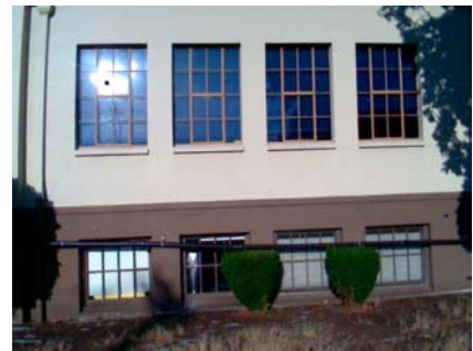
W Vertical Irregularity Secondary short columns ??
