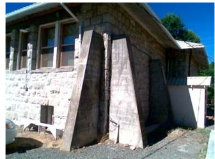
E Seismic Upgrade
