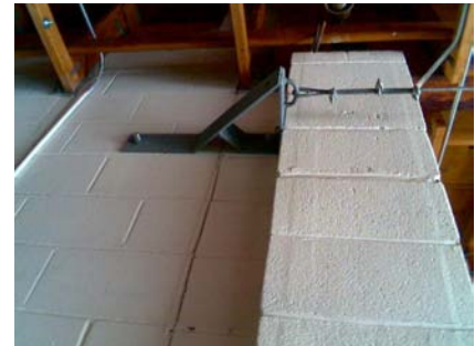
S Poor Condition Cables run throughout to hold the walls together.
