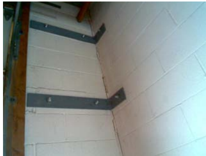
SE Poor Condition Straps were added later to keep the wall on the left from moving farther away from the wall on the right.
