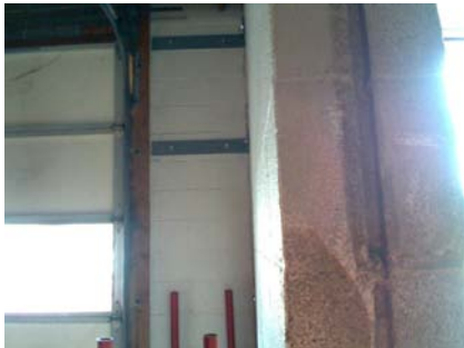
E Poor Condition light is showing through the edge of the RM1 wall just to the right of the door.
