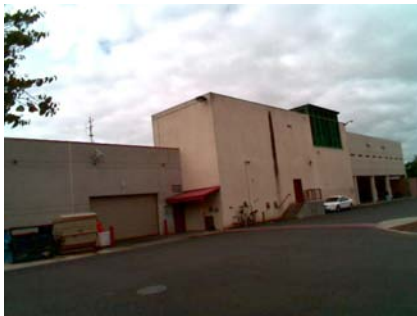
NE Elevation View
