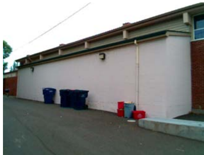
SE Secondary Structural Type RM1 side
