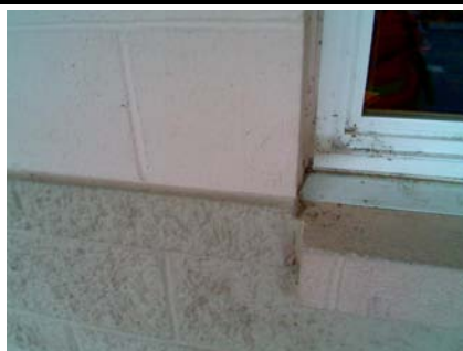
SW Primary Structural Type
