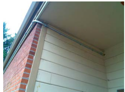
SW Primary Structural Type
