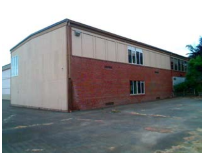
NE Elevation View
