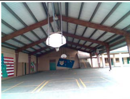
NE Elevation View
