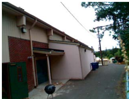
SW Secondary Structural Type
