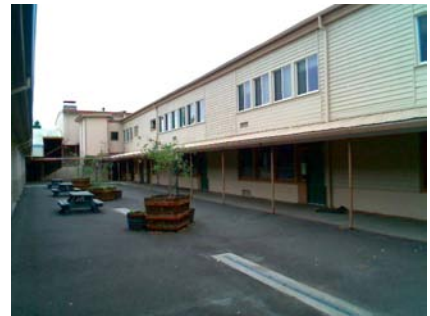
NE Elevation View
