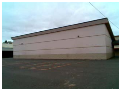
NE Elevation View
