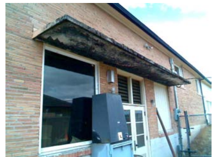
SE Falling Hazard Concrete overhang over door
