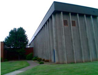
SW Vertical Irregularity Primary
