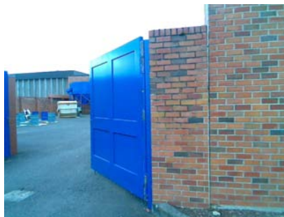
N Falling Hazard Wall disconnected at gap.
