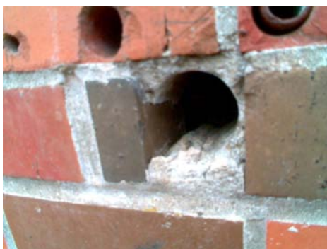
N Primary Structural Type Possible cavity wall, behind first layer of brick some concrete can be seen inside the hole
