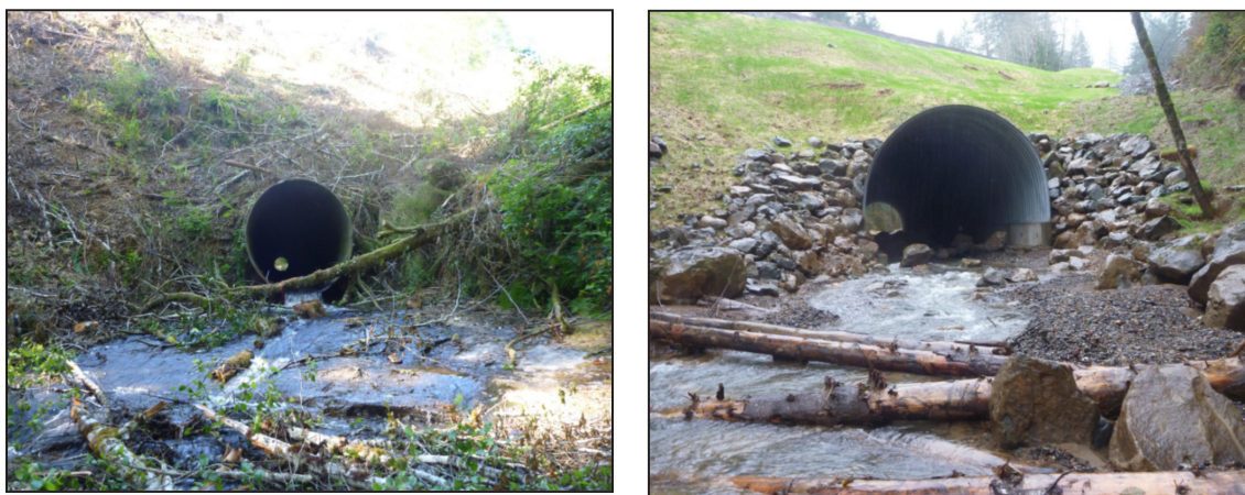
Figure 17. Undersized culvert with step blocked movement of Coho and Chinook to high quality upstream habitat (left). Culvert was removed and replaced with 26' wide arched steel set onto concrete footings (right), allowing natural stream habitat to be maintained through the 126' long passage. Source: CoosWA 2013
