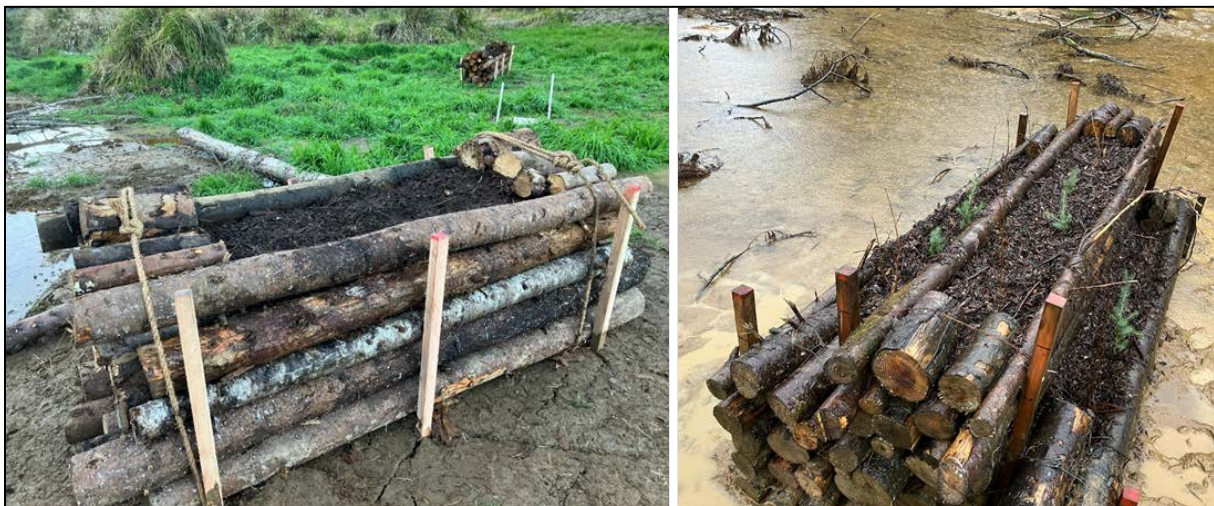
Figure 16. Examples of single chamber nurse crib (at left) and three-tiered nurse crib (at right) built in WZ1.
