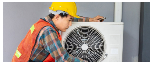
Technician installs a residential heat pump
