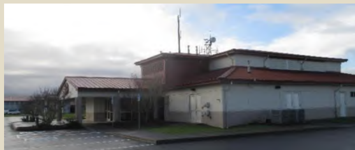
Emergency Operations Center, Building 7022
