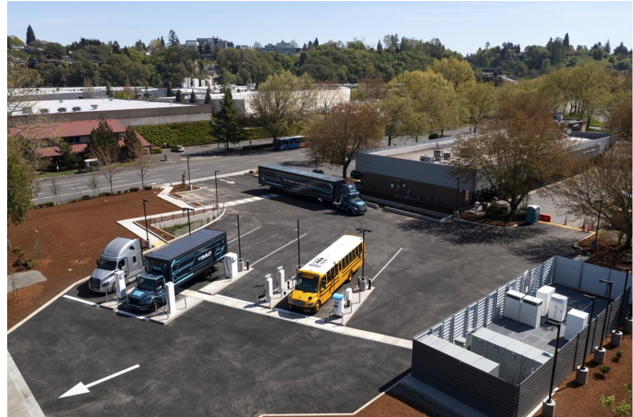
Electric Island – Daimler Trucks North America & Portland General Electric
