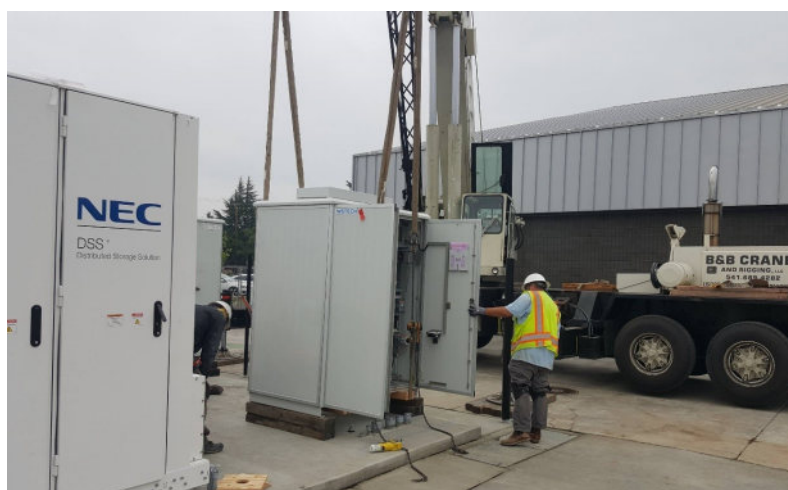
EWEB contractor installs back-up battery power system.
