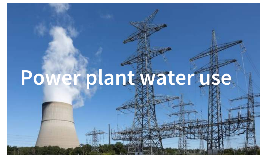
Steam rises above the cooling towers for a power plant. Google
