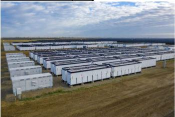
Over 90% of large-scale battery capacity in the U.S. uses lithium-ion chemistry<sup>3</sup>. Li-ion batteries have high energy density (compact size) and fast response, ideal for 1–4 hour storage needs.
