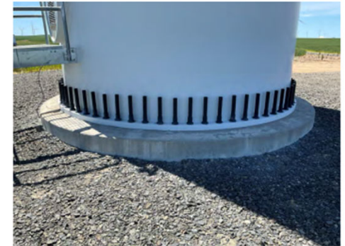
Figure 3-2 Example of low backfill condition
