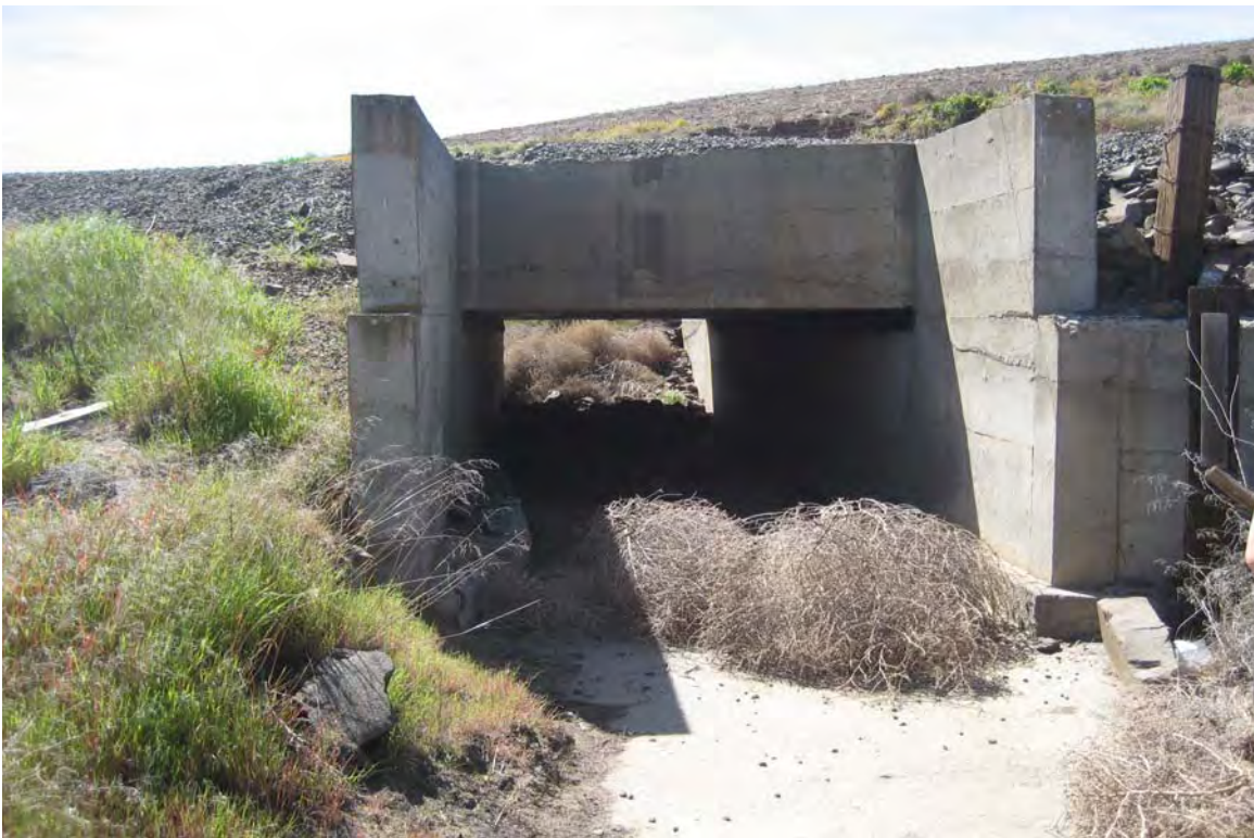
Photo Plate 4: Drainage D- Box Culvert
