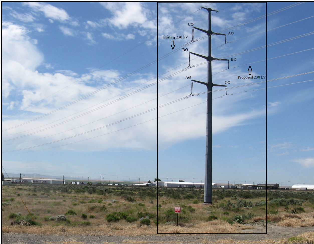
Figure 2-2: Proposed Hermiston to McNary 230 kV transmission line configuration.
