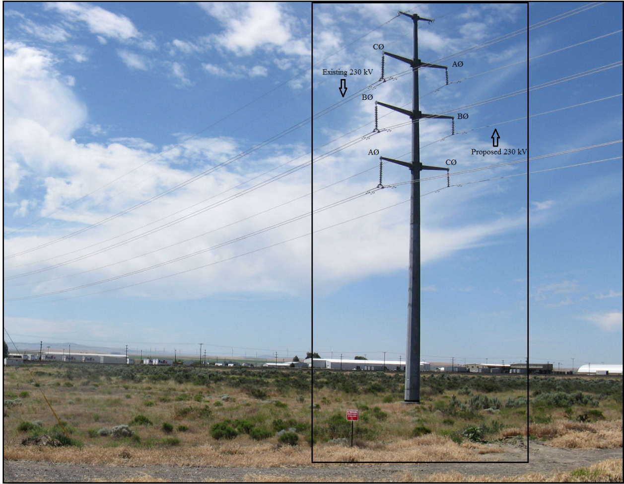
Figure AA-2 Proposed Hermiston to McNary 230-kV Transmission Line Configuration
