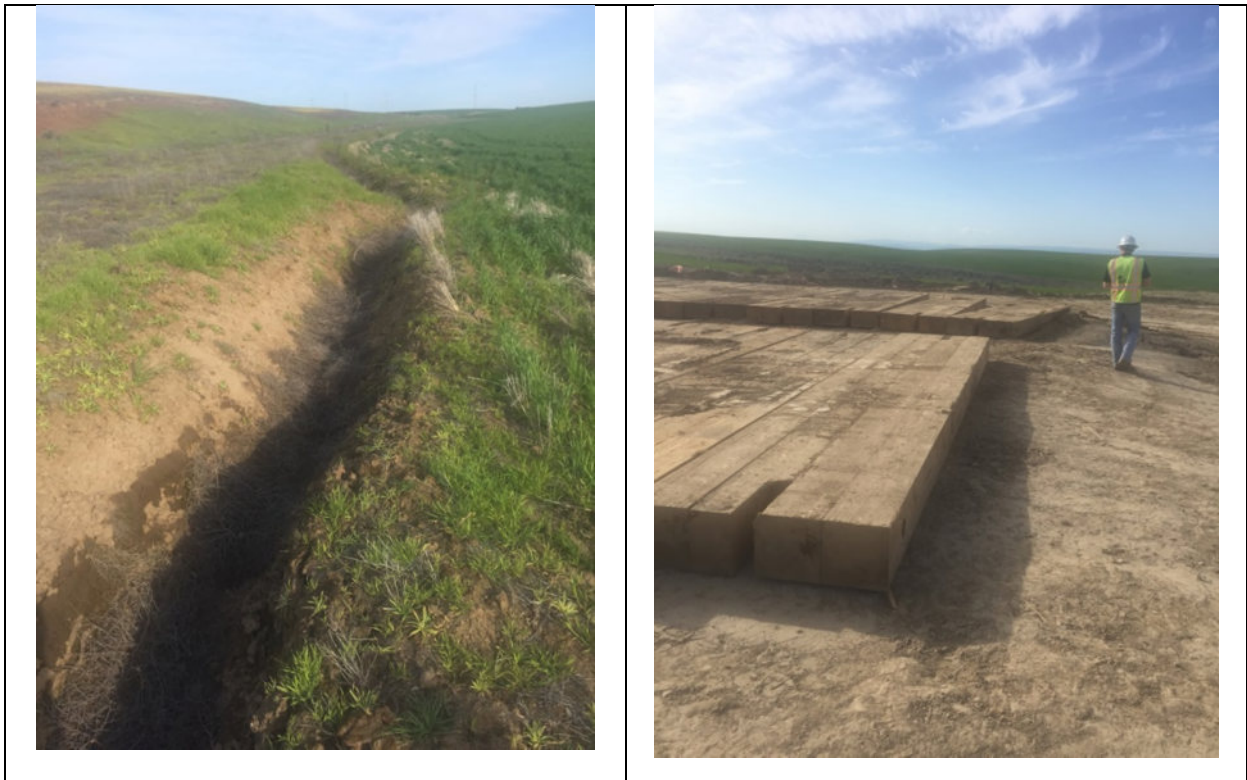
Figure 2. Stream crossing location (left) and typical crane mats (right)
