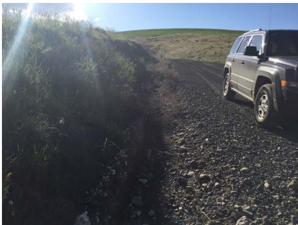
PP3021: Previously mapped roadside ditch that has been eliminated due to road maintenance activities (looking SW)
