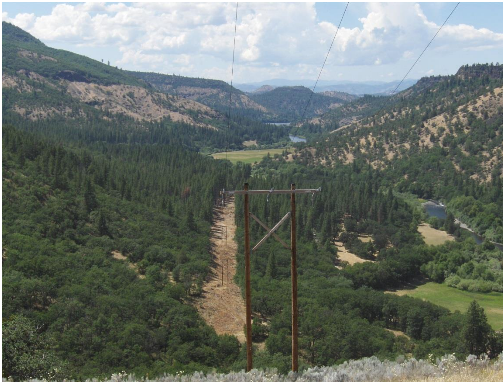
Figure 6.2. Line 4 in California following work (note the trees mid-span where the line is more than 100-feet off the ground).
