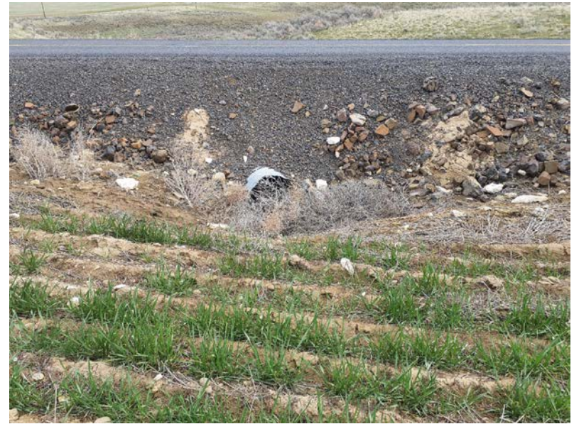
PhotoPoint_46. Photo Point. Looking E. Culvert inflow from plowed field full of tumbleweeds. 3/22/2022. Surveyor: SMF.
