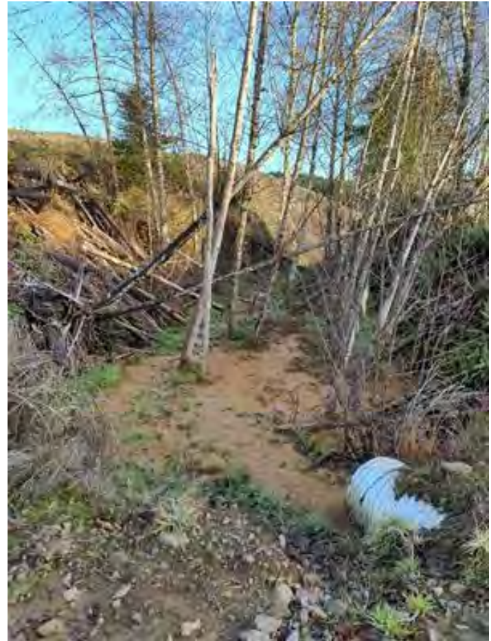
Photo 218. Culvert with sediment from the other side of the road after heavy rain. Ephemeral. Looking E. Taken: 12/20/2023. Lat/Long: 46.052154 -123.305456
